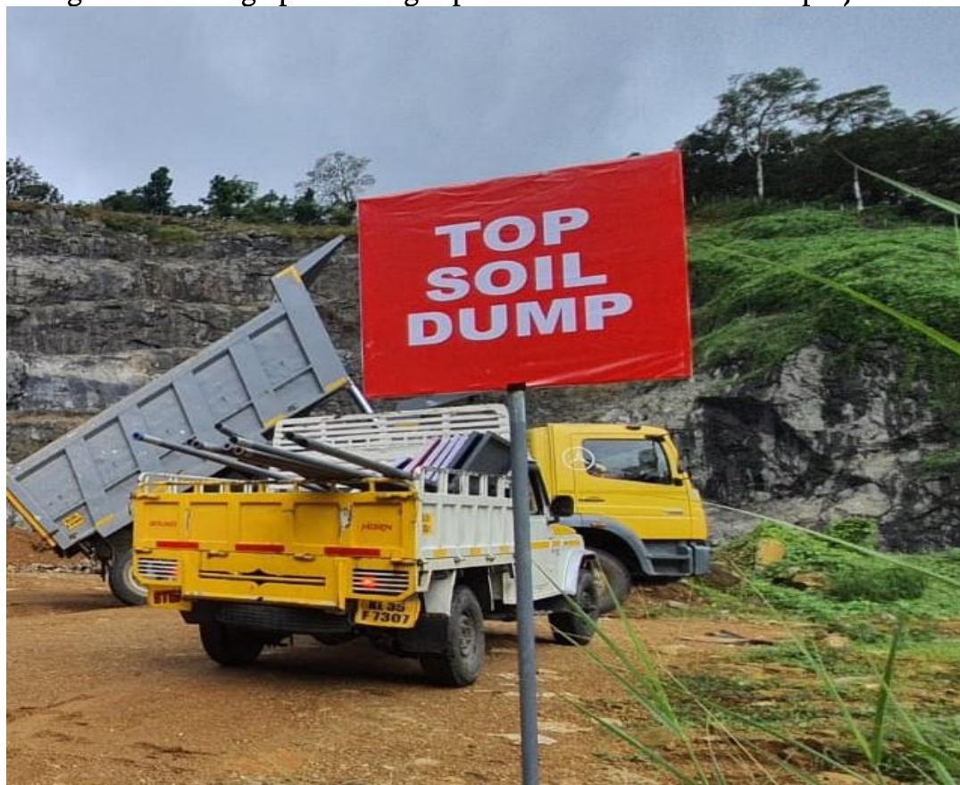
Figure I : Photograph showing top soil and overburden in the project site
