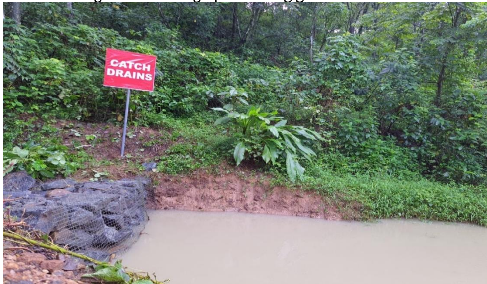
Figure-I3 Photograph showing garlad drains
