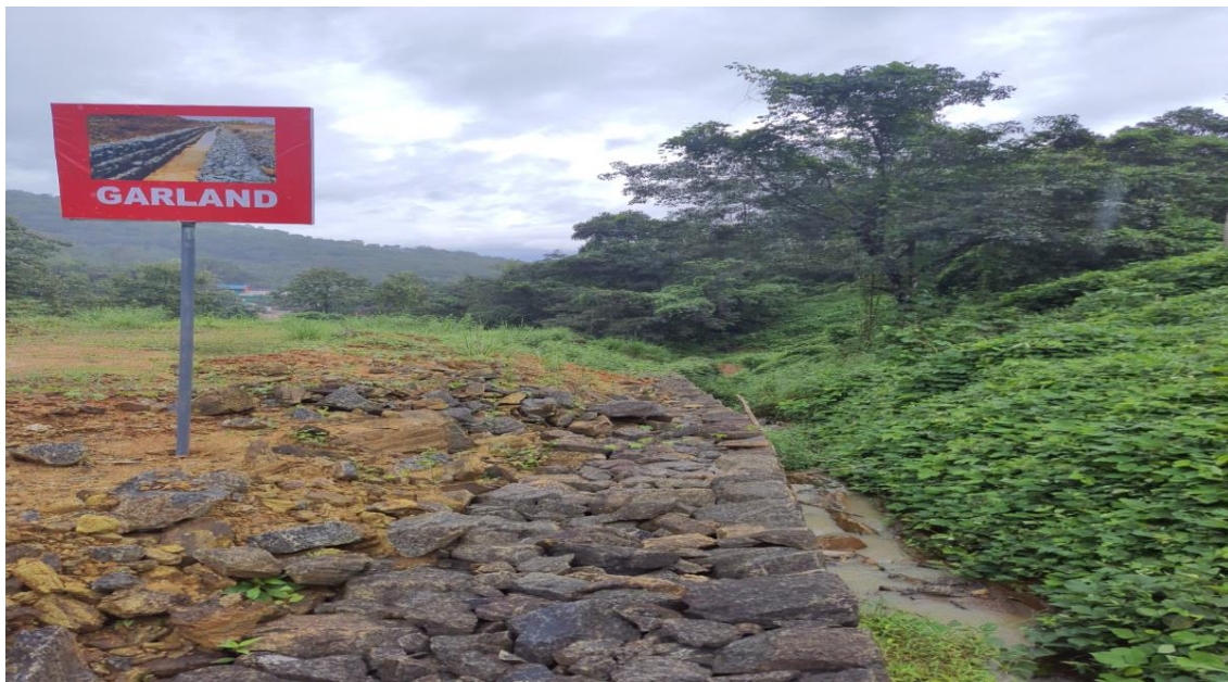
Figure 2 : Photographs showing garland drains
