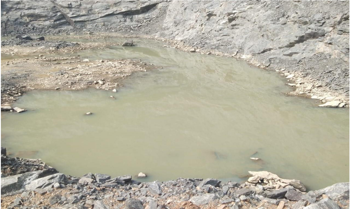
Figure 4 : Photograph of rain water harvesting pit
